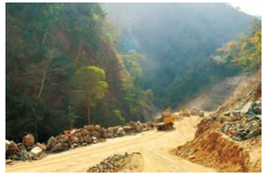
Fig. 6. Hydropower dam construction at Saw river (Mar. 4, 2014).
